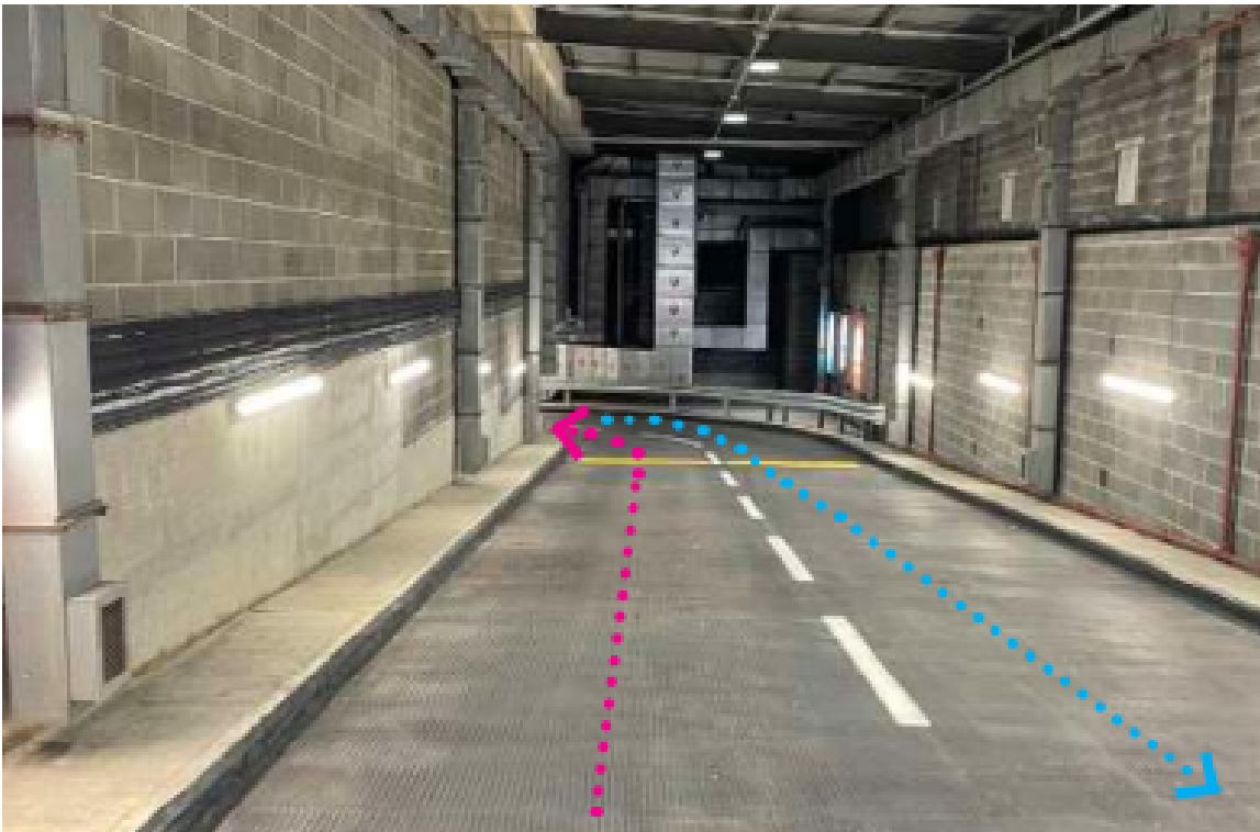
Image 7: Car Park ramp entry and exit
